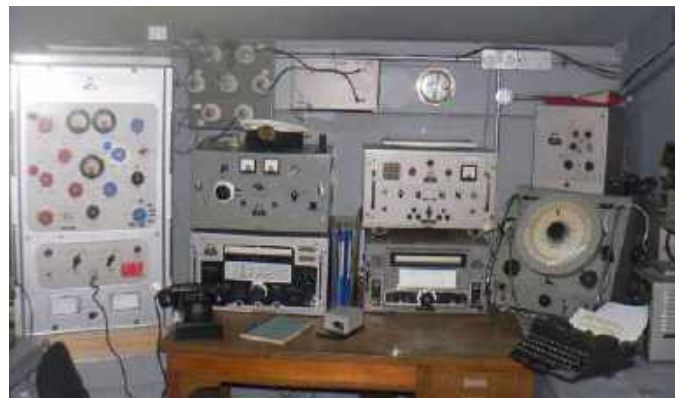
A typical Marconi radio room
